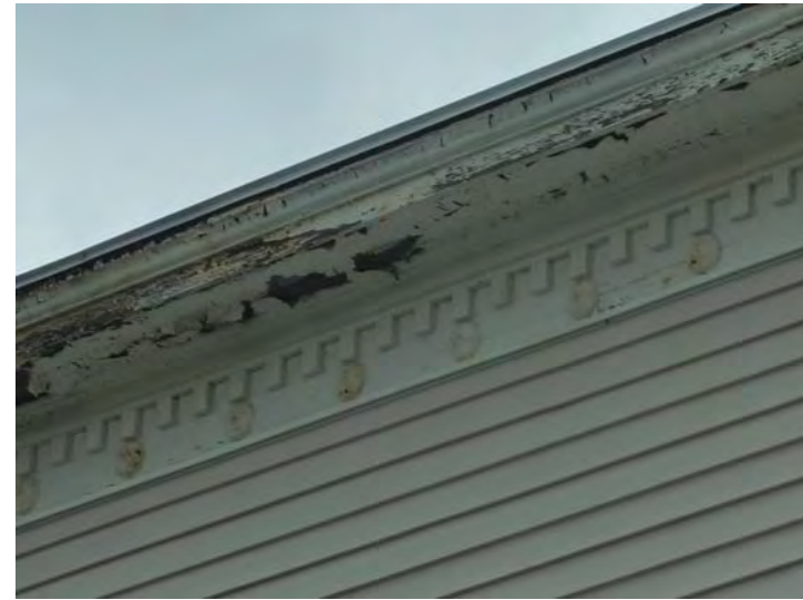
Typical soffit deterioration. Repairs and painting are shown in Year 1 and again late in the plan.
