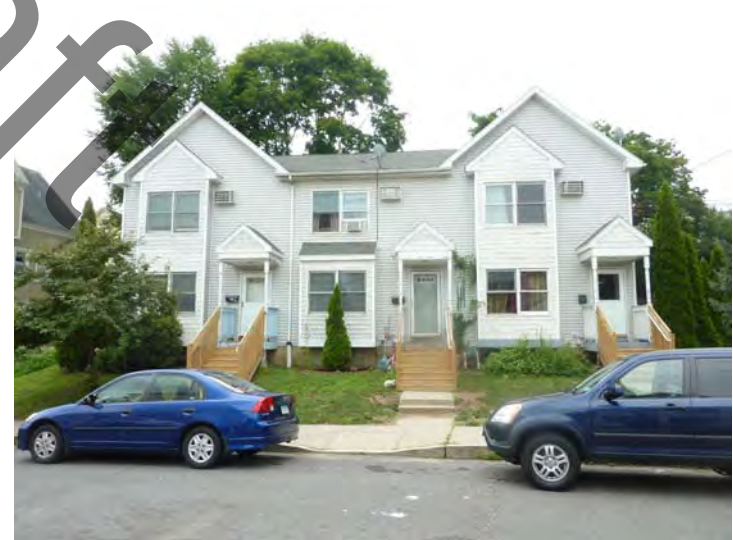
New wood stairs and steel handrails have recently been installed at 25-29 Lawrence.
