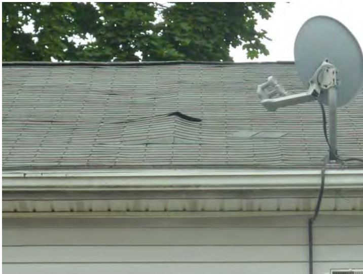
Localized asphalt shingle damage. Repairs are by management as needed. Replacement of asphalt shingle roofing and EPDM roofing is shown early in the plan.
