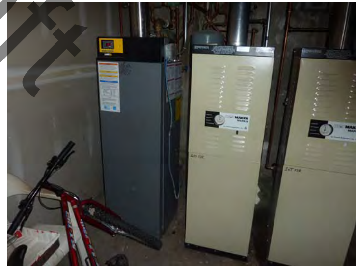
Typical gas-fired hot water boilers in basements serve each apartment. Replacement as needed is ongoing and overall replacement is shown for late in the plan.
